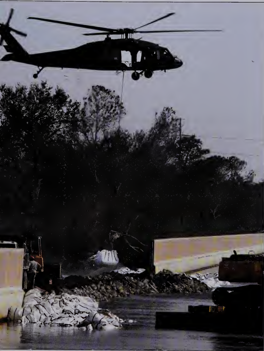
Plugging a breached floodwall, New Orleans
